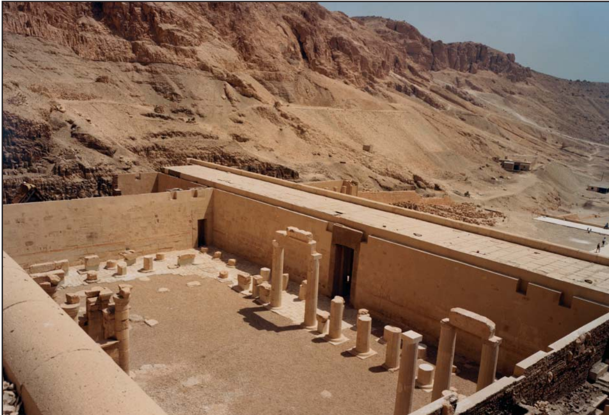
Temple of Hatshepsut. Upper Terrace. Festival Courtyard after restoration. Two restored architraves mark the two axes of the temple (Photo M. Jawornicki)
