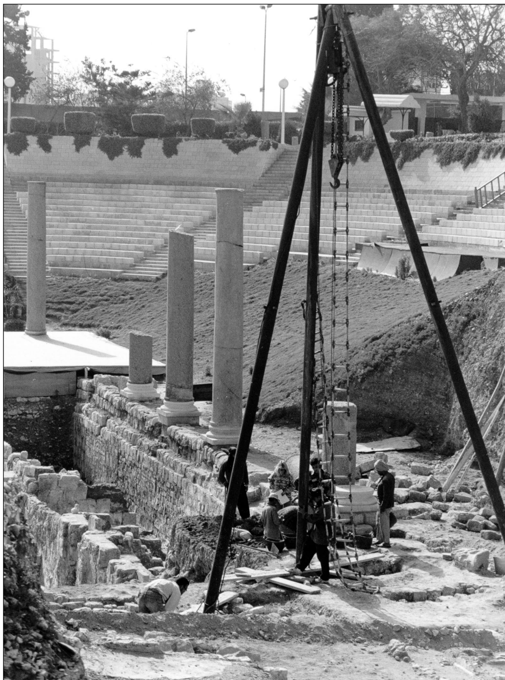
Fig. 6. Theater Portico. Raising another two columns discovered during excavations of the portico (Photo W. Kolqataj)
