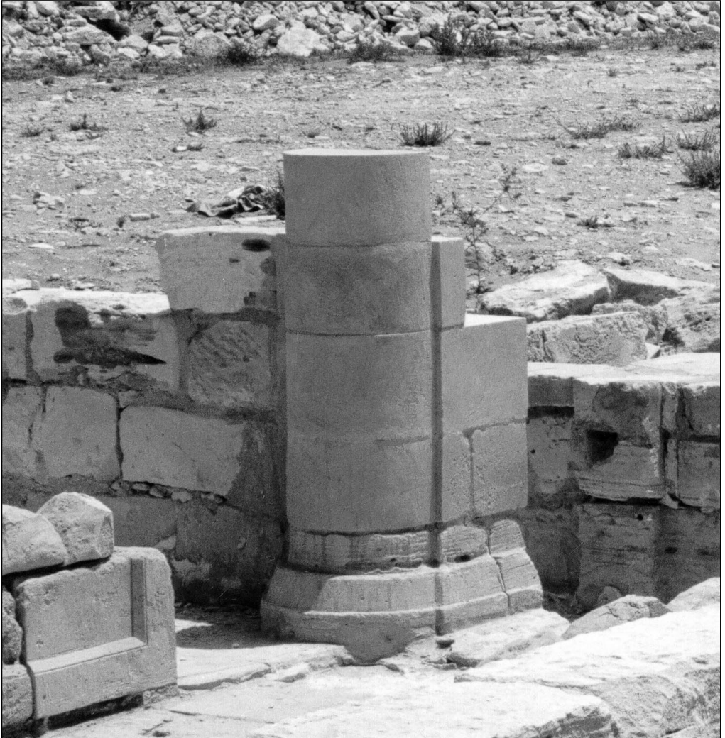
Fig. 11. Tomb-hypogeum T 6. A newly cut stone element in the aboveground mausoleum (Photo S. Medeksza)
