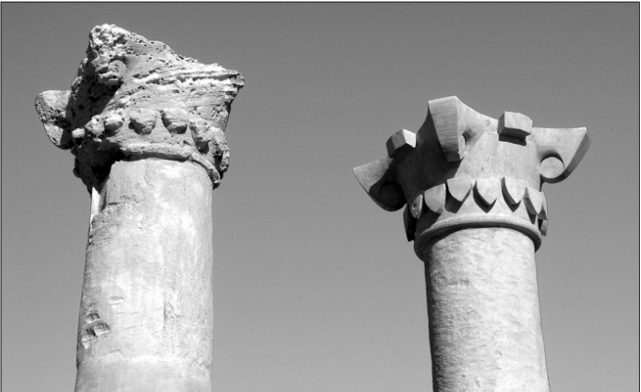
Fig. 10. Capitals from the commemorative monument in H21, after treatment (left) and reconstruction (right) in 2005 (Photo S. Medeksza)
