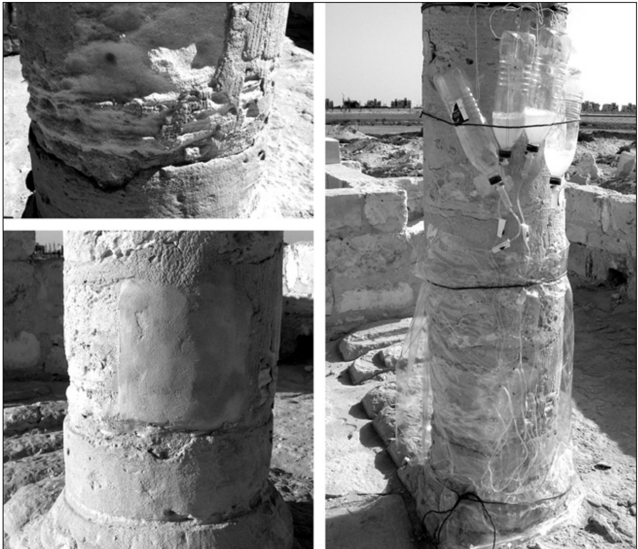
Fig. 12. Drum of a limestone column from H21, before (top left), during (right) and after trial conservation in 2005 (Photo P. Zambrzycki)
