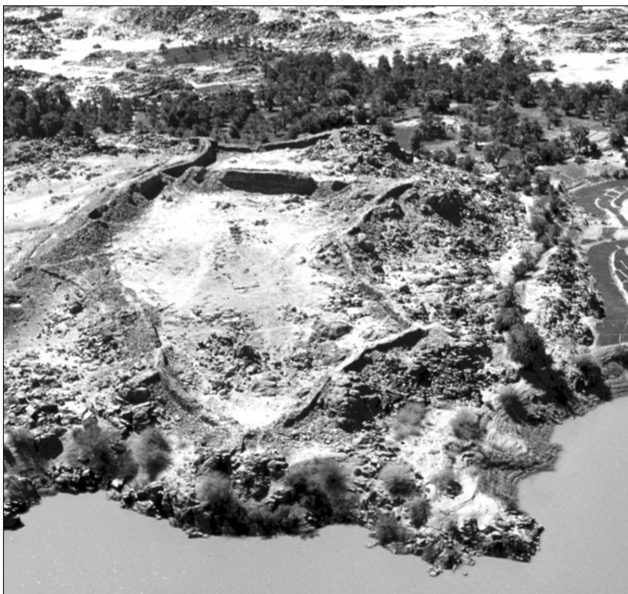
Fig. 1. Aerial view of the fortress of Dar el-Arab (=Swueqi el-Gharb), taken in February 2003 (Photo B. Żurawski)
