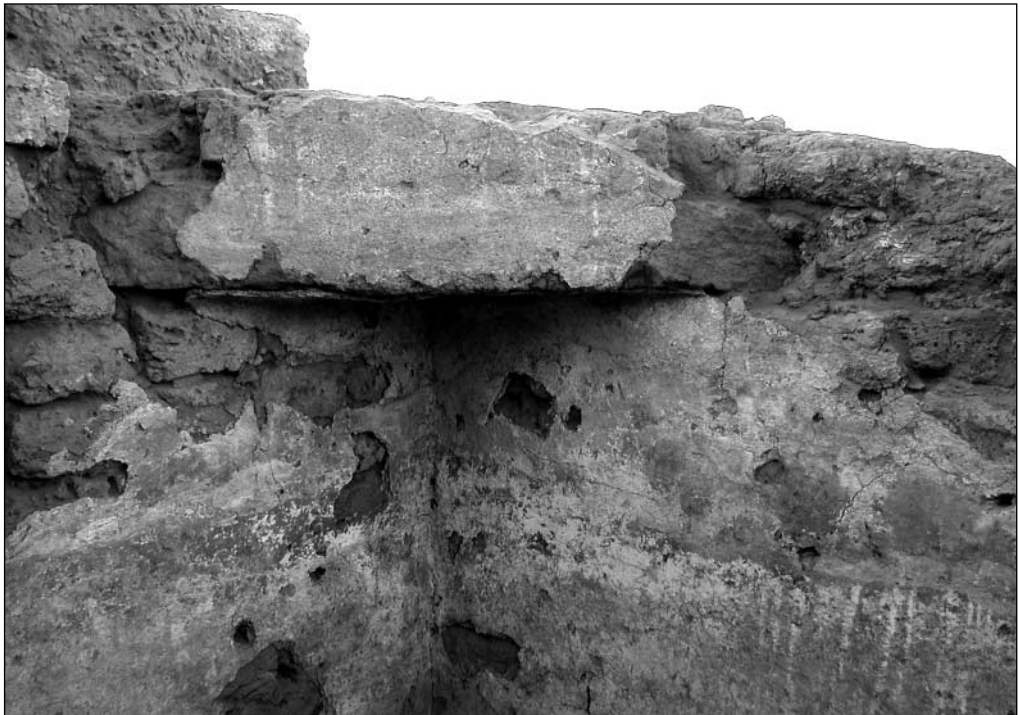
Fig. 9. Cruciform Building (B.III.1). Pendentive of the dome in the outer northeastern corner of the structure (Photo W. Godlewski)
