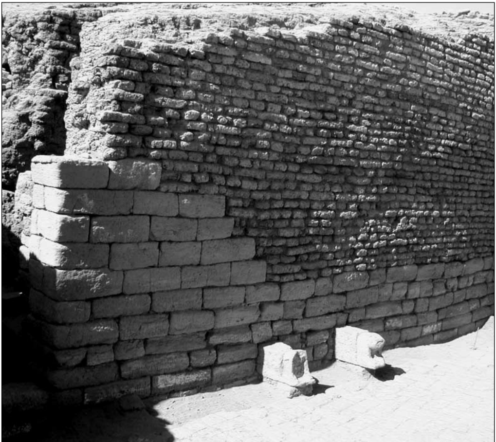
Fig. 3. Site SWN. Building B.I, south wall (staircase façade) (Photo W. Godlewski)
