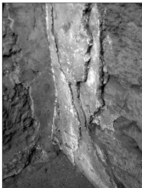
Fig. 2. Stratigraphy of lime plaster coatings preserved in the northern arm (Photo D. Zielińska)
